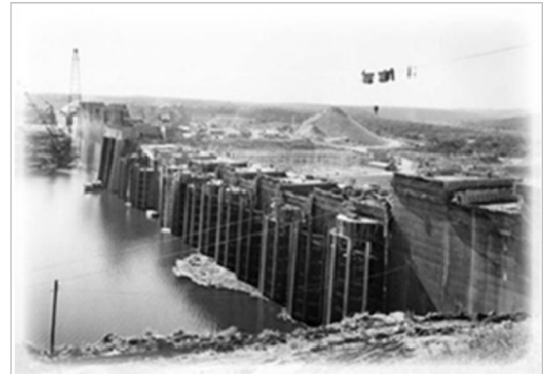
(Mansfield Dam photo taken 11/1/40 and is courtesy of LCRA Corporate Archives)
