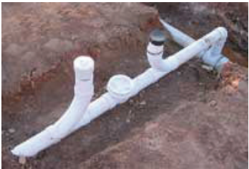
Pop Off Valve and Check Valve
